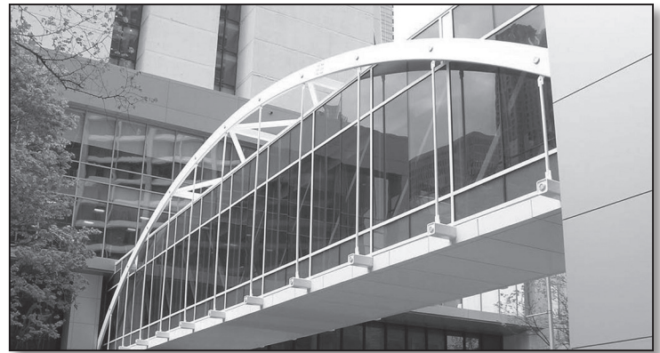
Pedestrian skybridge at the Atlanta Hilton connecting the Atlanta Hilton and the Atlanta Marriott Marquis
