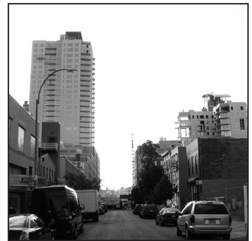
New waterfront construction, 2009. Photo: Sharon Zukin.
